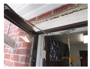
**Figure 17 Degrading Lintels**
